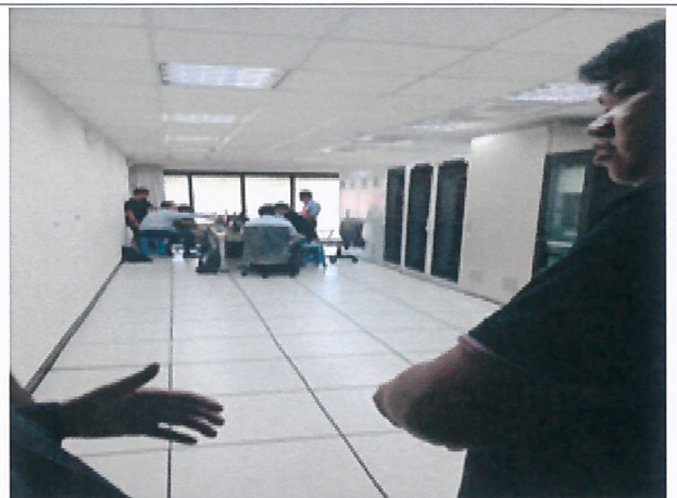
Onshore S/S Control Room
